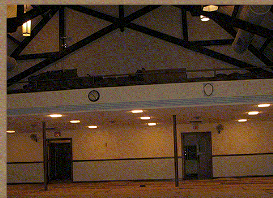
Original upper level balcony removed
