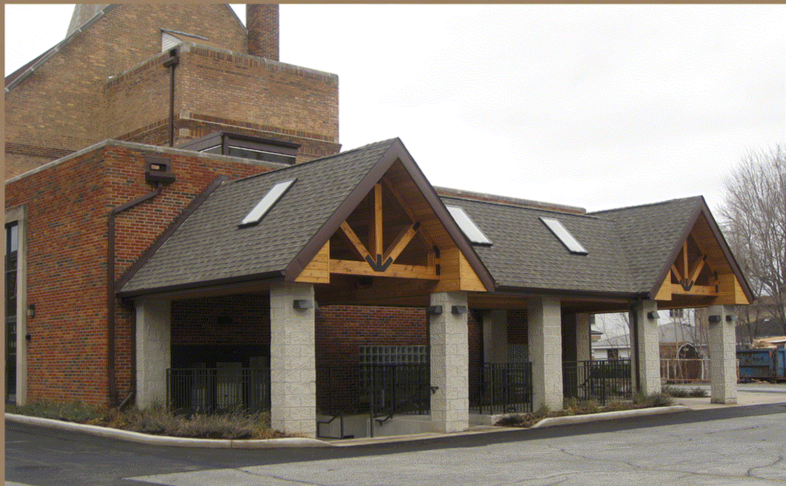
New covered East addition
